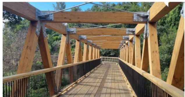
Timber Structure Bracing
