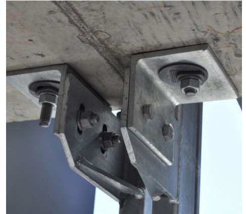
Upper connection: OrbiPlate™ and Ramset™ TruBolts
