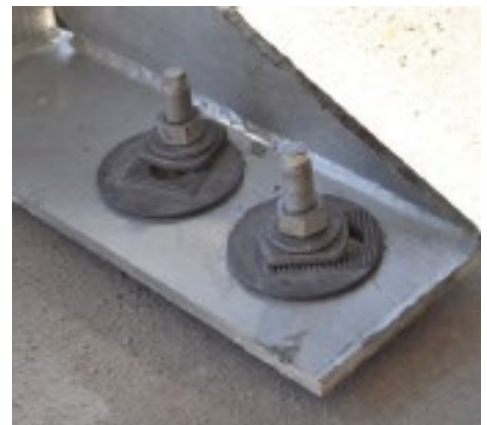
Lower Connection: OrbiPlate™ and Ramset™ ChemSet™ 502
