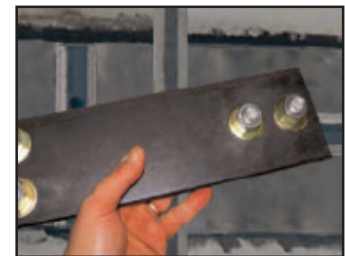
Figure 5 connection plate being installed
