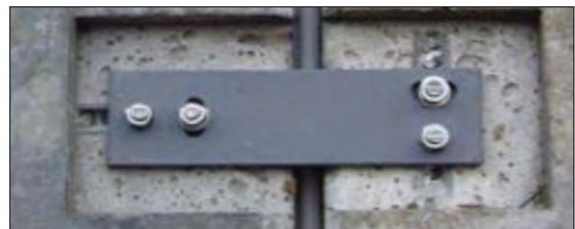
Figure 6 cast in toothed channel in finished construction
