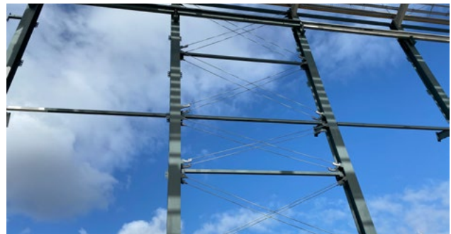
Structural Steel Structure Bracing
