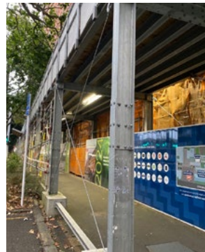
Temporary Work / Platform Bracing
