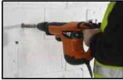
1. Drill hole to specified diameter and depth with Ramset™ DynaDrill™
